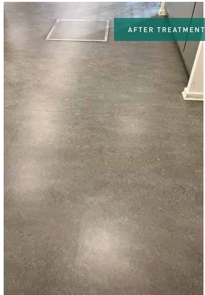
Corridor areas at a district heating plant - Treated with PUR Intensive Cleaner, sanded and finished with 2 coats of PUR Floor Sealer
