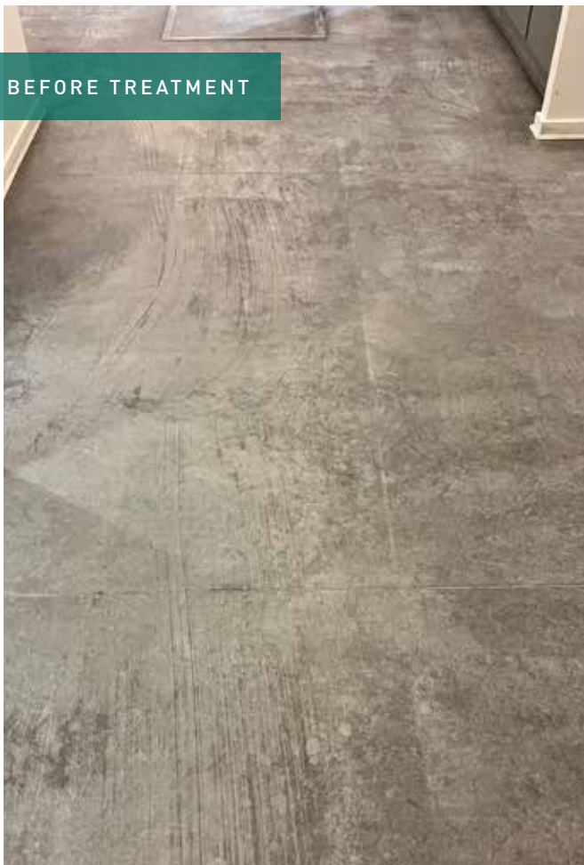
Corridor areas at a district heating plant - Treated with PUR Intensive Cleaner, sanded and finished with 2 coats of PUR Floor Sealer
